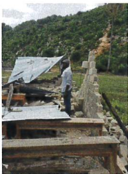
The remains of one of the Moravian Buildings in Haiti
